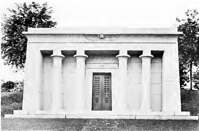
Subject 8979½. Permanency being the basic reason for mausoleums, the massiveness of the Egyptian architecture is particularly adaptable to that enduring construction. Of Barre Granite. Erected for the Estate of Wm. Patterson at Oak Park Cemetery, Newcastle, Pa.
